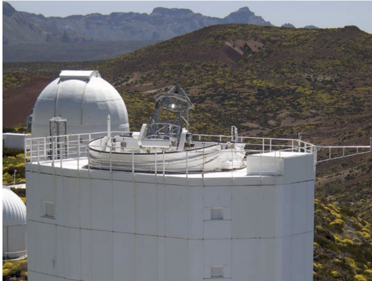
Figure 1. GREGOR telescope facing the Sun, with open dome. The dome on the left of the picture is from the ESA optical ground station (OGS). The bright spot inside the telescope structure is the reflection of the incident sunlight off the field stop.
