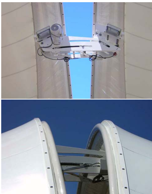
Fig. 7 (online colour at: www.an-journal.org ) Partial view of the nearly closed GREGOR dome. Motorized clamps pull and lock the two halves together, to provide optimum strain to the cloth. Top : inside view, bottom : outside view.
